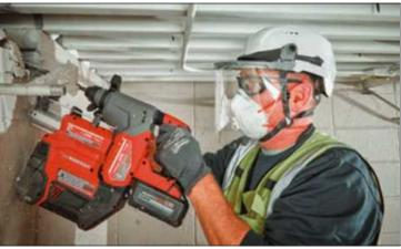
AVAILABLE WITH adjustable chin straps, ear protection and face shields, construction safety helmets are gaining popularity on today's jobsites. Photo credit: The Construction User
